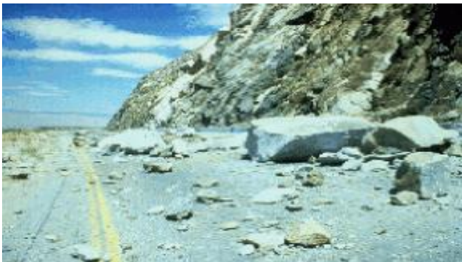
Failure of a hill slope
