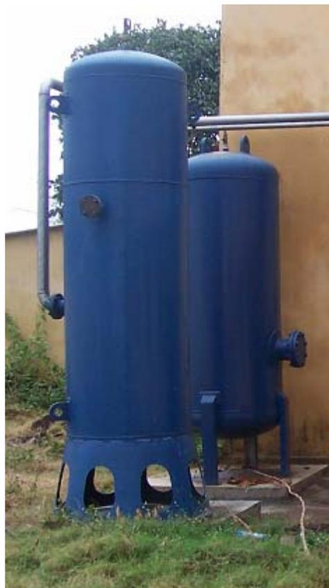
**Figure 5.11:** Photograph of 37 kW compressor receivers.
