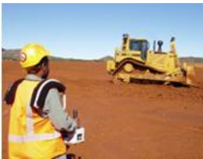
Fig.6.1 Dozer being remotely controlled.
