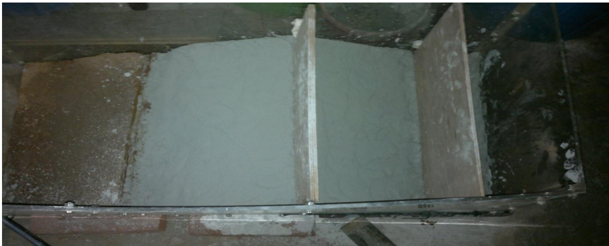
Fig.4.27 Making Of The Second Stage Dyke
