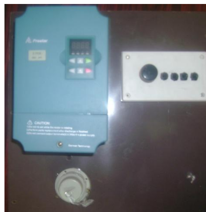
Fig: 10. Variable Frequency Drive with its circuit board.
