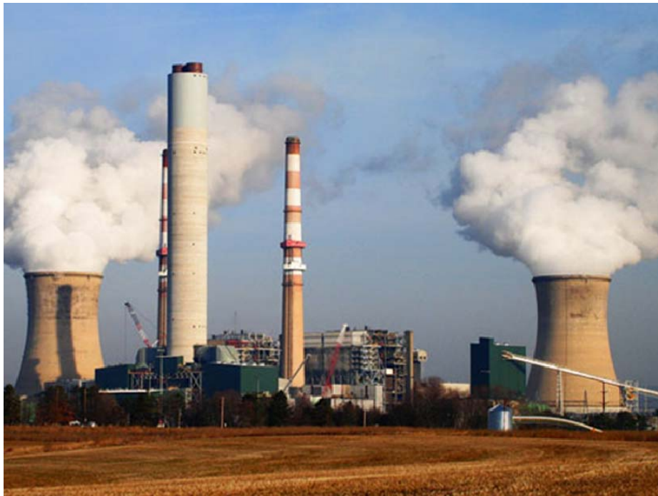
Fig. 1: Self-supporting Steel Chimney (ref. http://www.comdynam.com/ )
