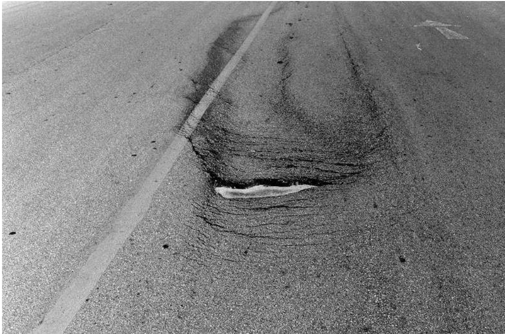
Figure 1.1: Slippage Crack ( http://www.surface-engineering.net )
