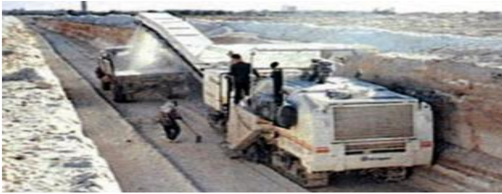
Fig-2.4 trenching by surface miner
