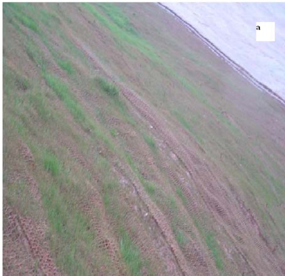
Figure 3 (a) Coir Matting on dump slope
