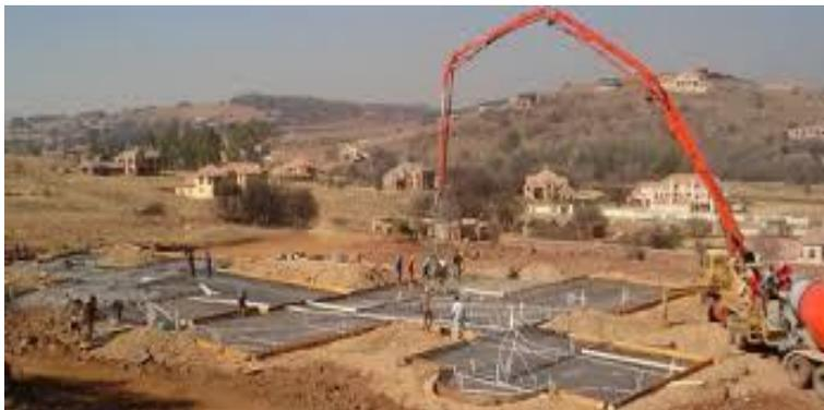
Figure 1: Construction of Raft Foundation
