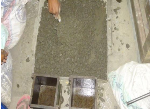
a) Mixing of concrete ingredients
