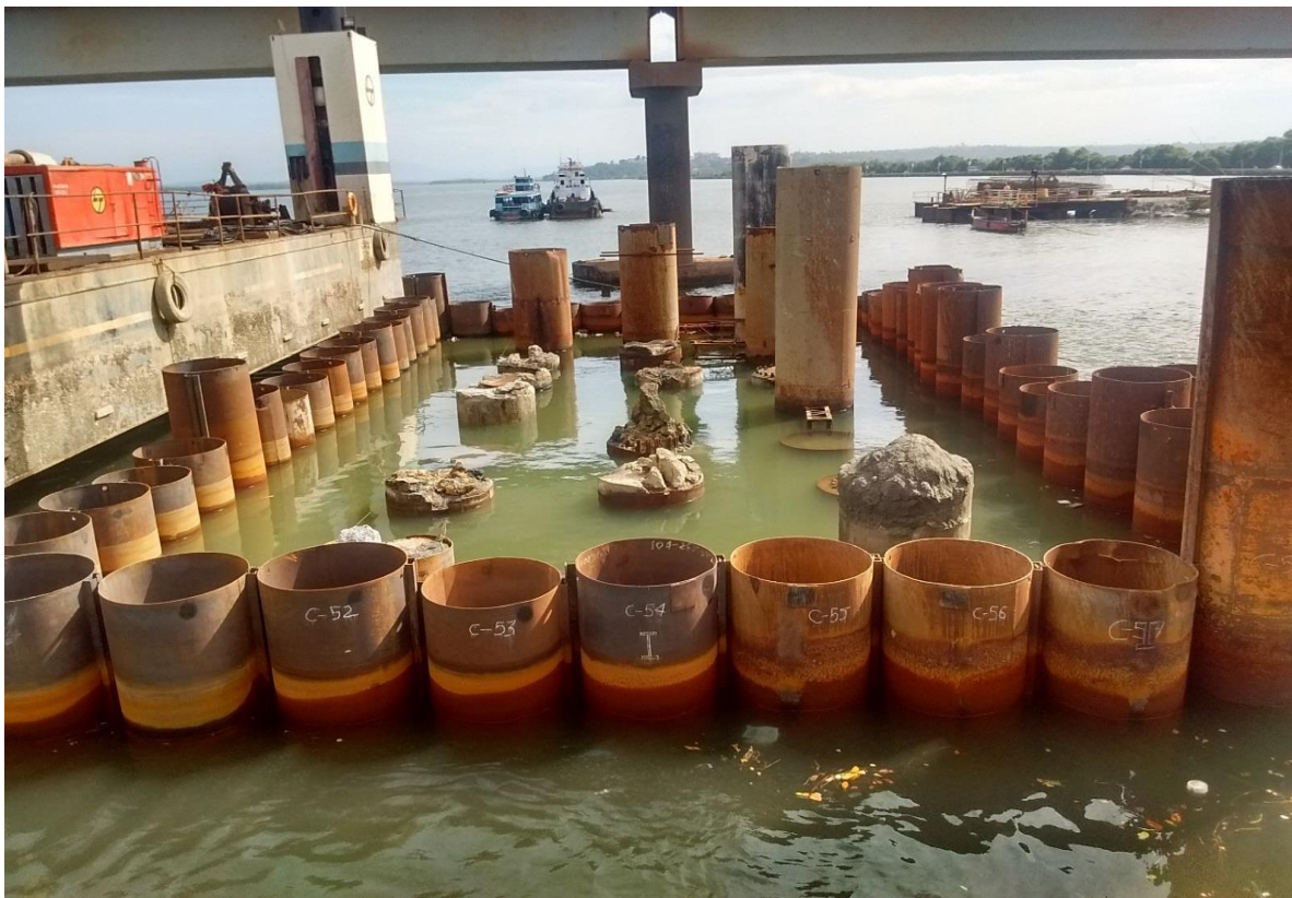
Fig 3.2 : Cofferdam at P-22, MRCSB Project
