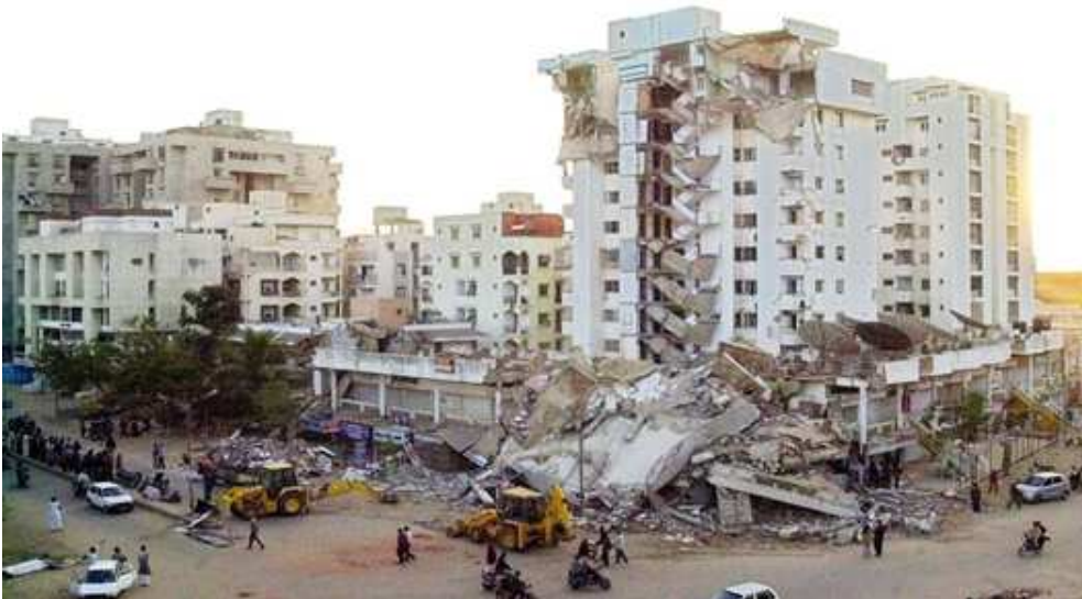
Figure 1.1: Picture of Bhuj Earthquake damaged building, Gujrat, India ( www.googlelet.com )
