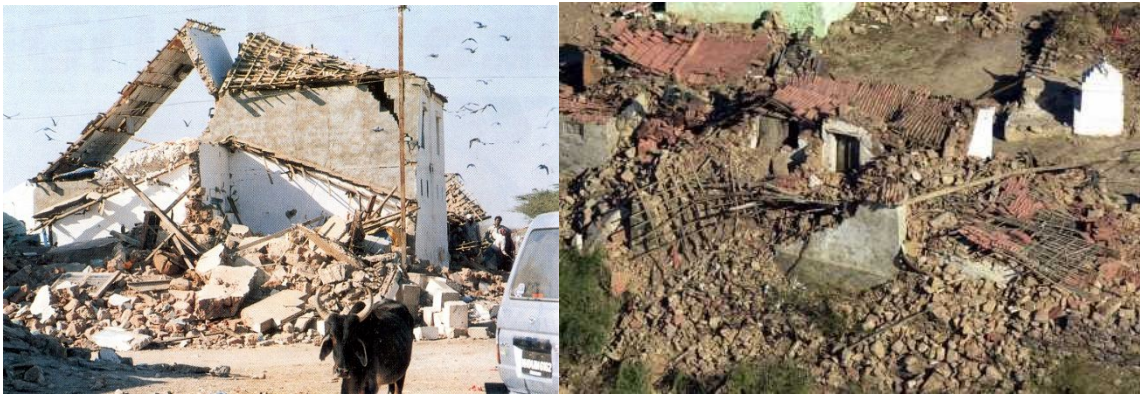
Fig. 6.1: Bhuj earthquake damage to URM, 2001
