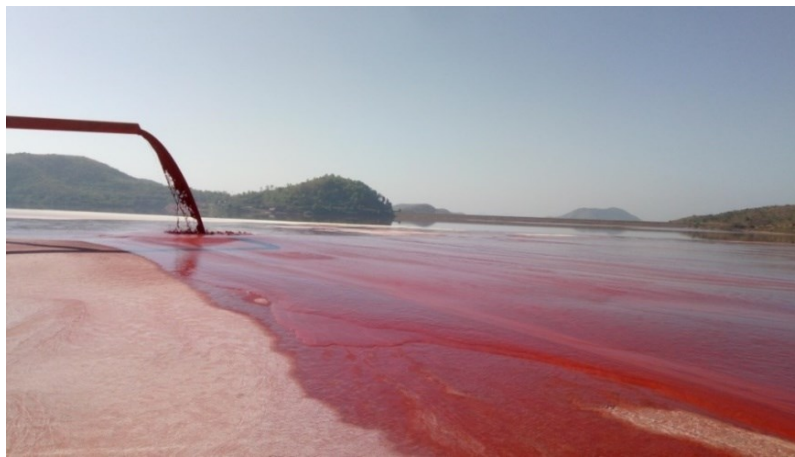
Figure 1.3. Slurry disposal system of NALCO, Damanjodi (photo by S. Alam)
