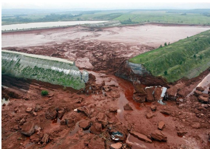
Figure 1.6. Red mud pond dike failure in Ajka, Hungary
